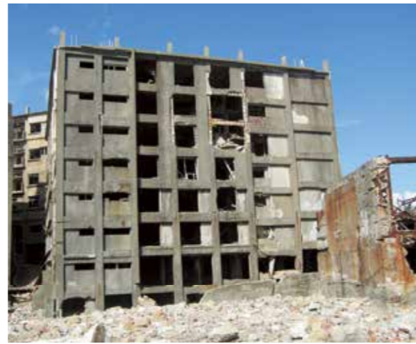
No. 30 and No. 31 Apartment Buildings
