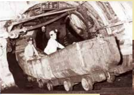
◀ Carrying coal waste out of the mine. ▶ Pushing a fully loaded 'coal tub' to the main mining cart tracks.
